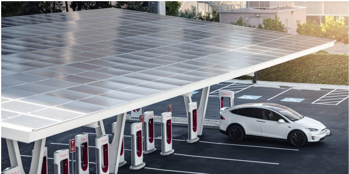
Obrázok 32 Tesla parking port V3 Supercharger station (250 kW)
